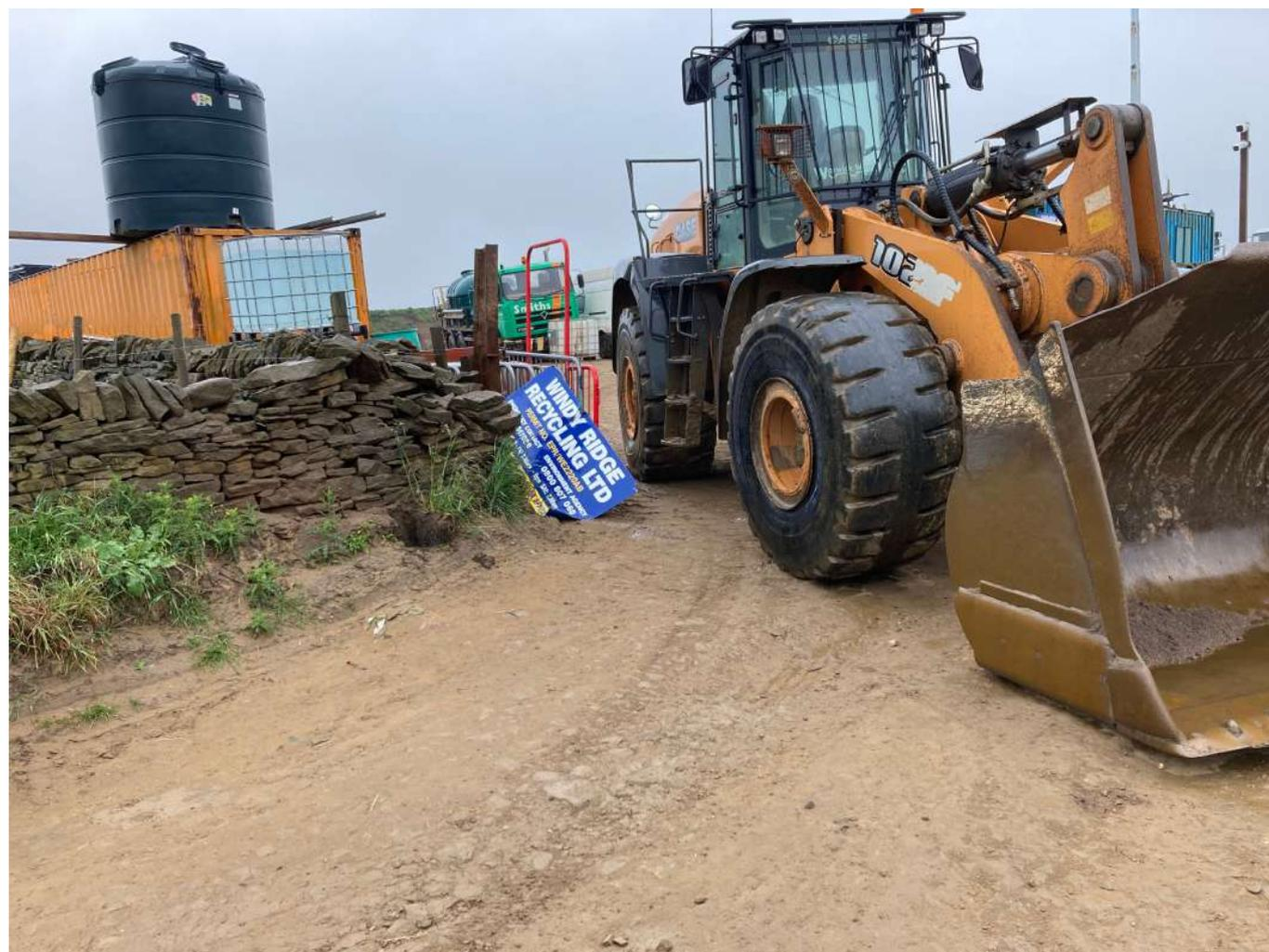
Further along the Bridleway there is evidence of major excavation taking the road surface several metres below the original level, removing the verges and leaving what looks to be unstable dry stone walls
