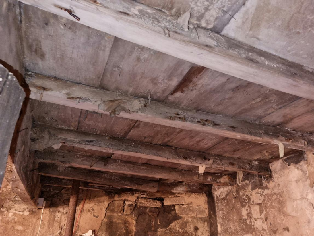
Flooring needing repair/replacing.
