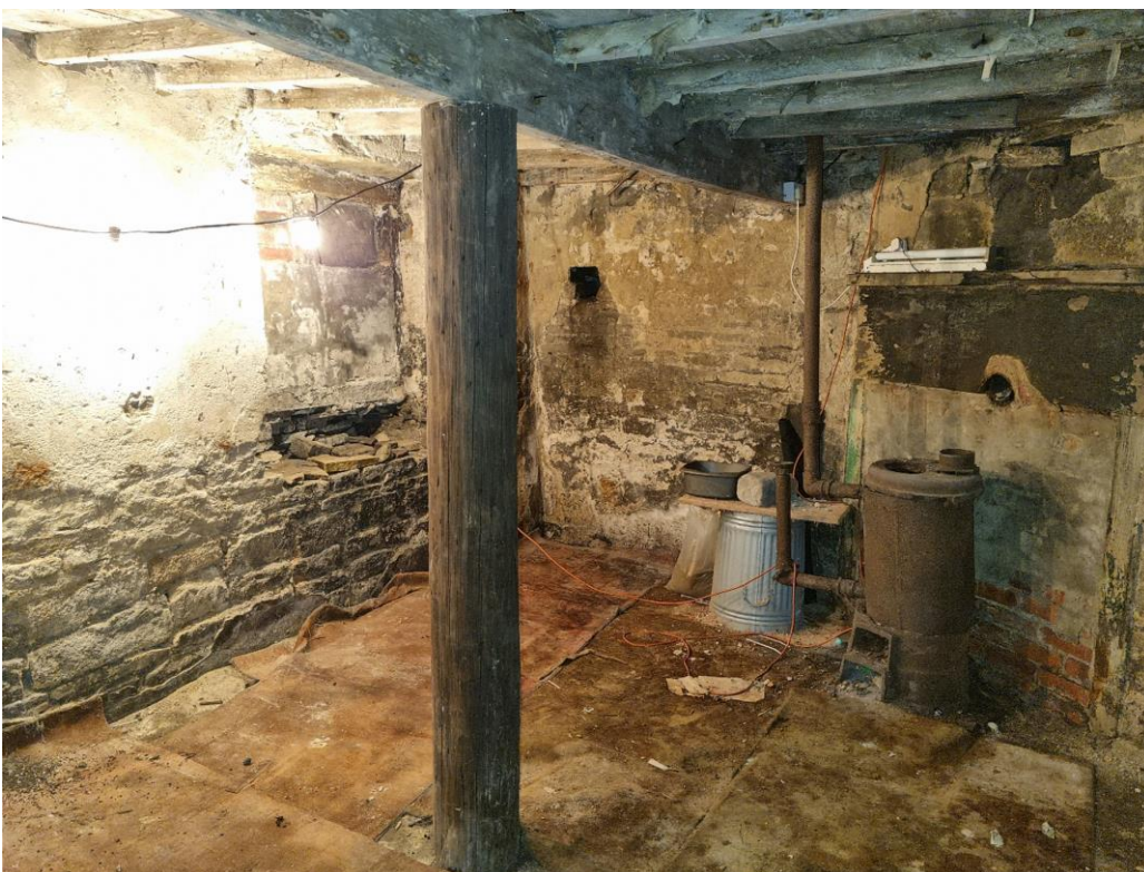
Telegraph pole in cellar supporting the floor. Future plans include converting the cellar area into a practice space for individuals, and for lessons.
