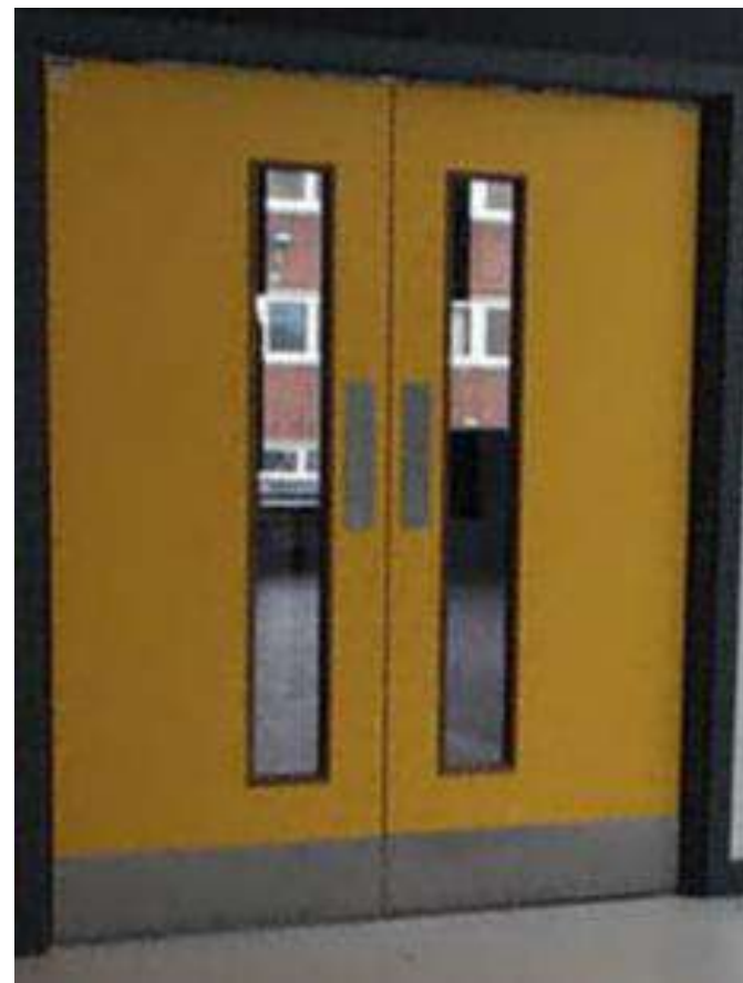
INTERNAL TIMBER DOUBLE DOORSET TO GROUND FLOOR HALL WITH PAINT FINISH – COLOURS TBC
